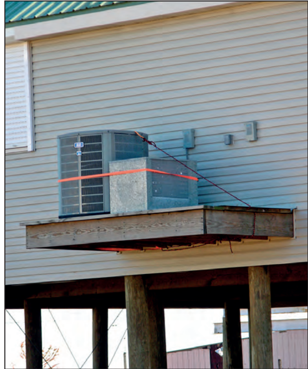
Figure 3-2. Air conditioning compressor elevated on a cantilevered platform.
